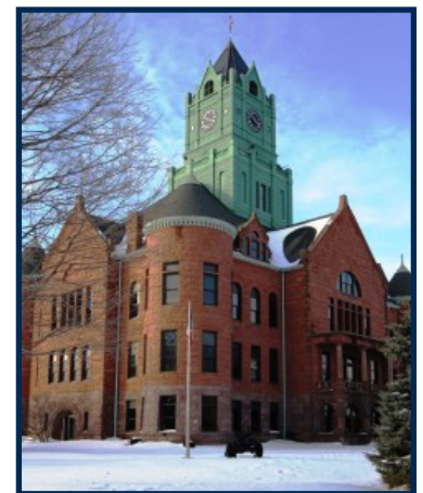
Clinton County Courthouse
